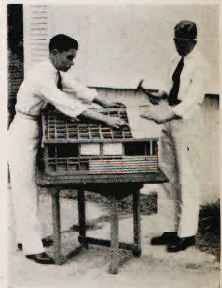
Laying the roof.
