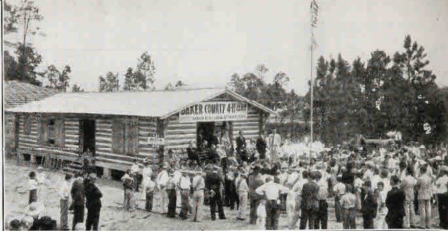
A public address system carried the program to 3,000 people attending the dedication of this fine club building. Note unfinished livestock pavilion at left rear.
