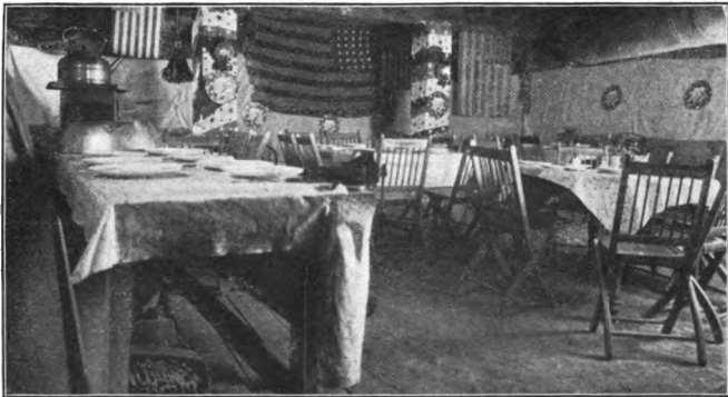
FIG. 140. The Workshop of Cottage Hill School. Workbenches used for Lunch Counters
