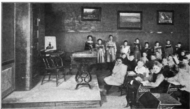
FIG. 59. A Room in the Seward Consolidated School
